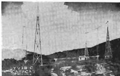
Here we have the antenna equipment of Radiodifusora Venezuela, YV3RC, Caracas, which transmits on a frequency of 6.150 megacycles. YV3RC is quite generally received throughout North America.
